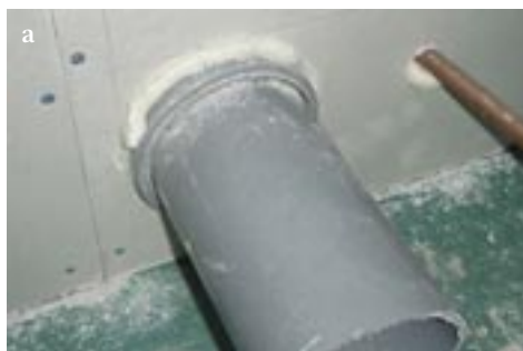
Figure 15 (a) and (b) Good sealing around services penetrations.
