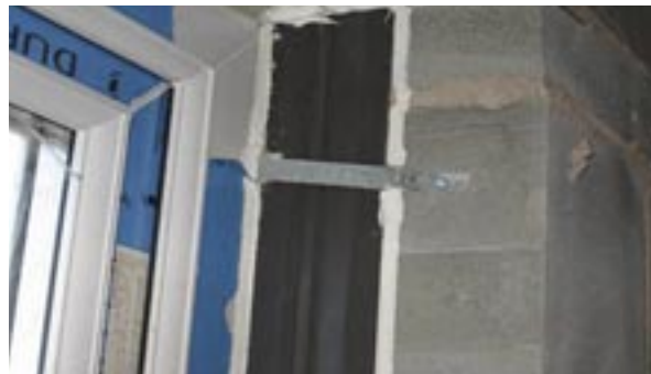
Figure 12 Proprietary cavity seal at the window reveals.
