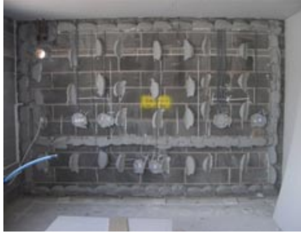
Figure 17 Blockwork wall providing air barrier: dry lining can now be fixed.
